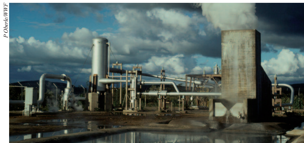
Olkaria II geothermal plant in Kenya.
